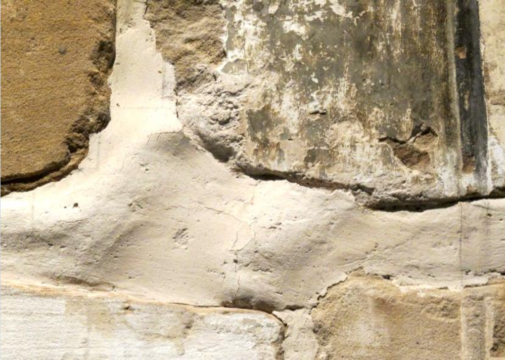
Salt crystallization & Flaking of stone artefacts
