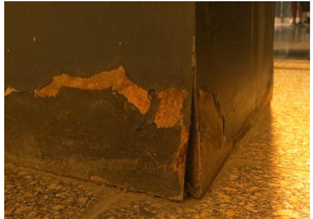
Metal corrosion bronze and cooper alloys
